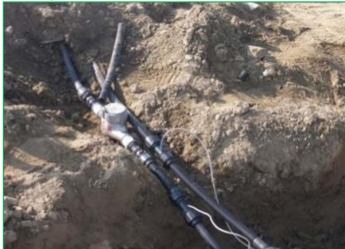
Two pipes subsoil heating system
